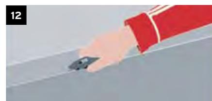
**12.** Using a sharp knife or Araseur trim the carpet to fit against perimeter walls.
