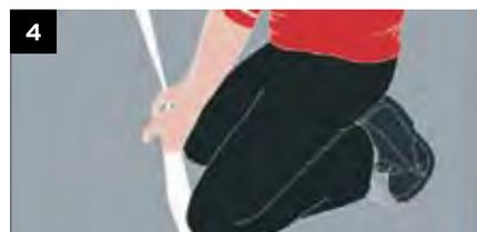
**4.** Measure and cut the second piece from the roll. Position the second piece with the edge overlapping the first by approximately 5cm and mark a guide line on the floor with a pencil at the next seaming edge.
