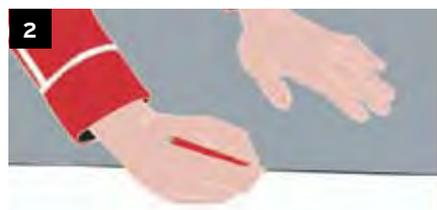
**2.** Run a pencil along the inner edge of the flooring making a guide line on the floor for the application of adhesive.
