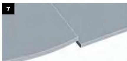
**8.** Fold back both edges by half the width of the carpet taking care not to disturb the positioning of the carpet. Apply the recommended adhesive to the subfloor, then re-position the first piece of carpet and roll with a 68kg flooring roller to ensure overall contact with the adhesive.
