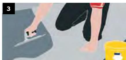
**3.** Fold the sheet half way back taking care not to disturb the positioning of the flooring. Apply the recommended adhesive onto the subfloor, from the wall to within 20cm of the guide line. Replace the carpet carefully and accurately back into position and roll with a 68kg flooring roller to ensure overall contact with the adhesive. Repeat for the other half of the sheet.
