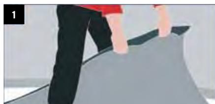
**1.** Wherever possible lay the carpet down the length of the room to minimise the number of joints. Avoid joints in doorways and high density traffic areas. Measure the length of the room, and cut the first piece from the roll allowing an additional 75mm for trimming. Ensure an allowance is made for doorways, alcoves and any irregularities of the walls. Starting at the corner furthest from the door, lay the first piece into position lapping up the walls at both ends for sufficient trimming.
