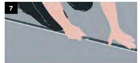
**7.** Position a straight edge along the middle of the overlap and cut through both pieces of carpet with a sharp knife and remove the surplus. Fold back the seam edges and apply adhesive onto the subfloor with a notched spreader. Re-lay the carpet and roll with a 68kg flooring roller to ensure overall contact with the adhesive.
